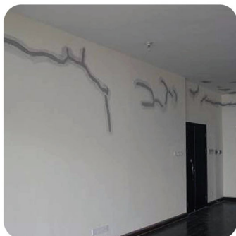
Cracks & Repair Works
